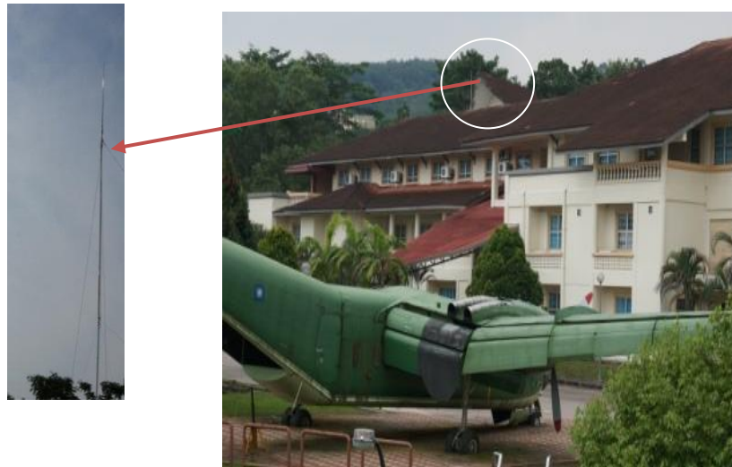
Figure 3: AIS antenna installed at P23, Faculty Mechanical Engineering, Universiti Teknologi Malaysia
