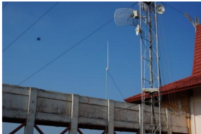
Figure 9: AIS antenna installed on top of a building structure of Politeknik Negeri Batam
